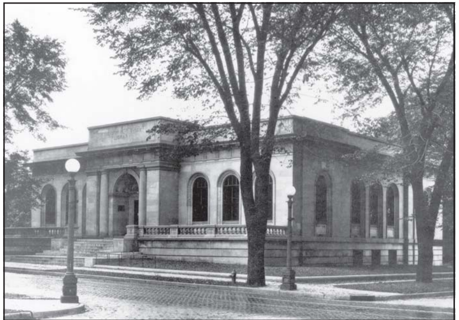
The Urbana Free Library, previously named the Samuel T. Busey Library, circa 1918
